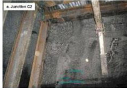
Figure 5. The exposed roof Junction C 2 [22]
